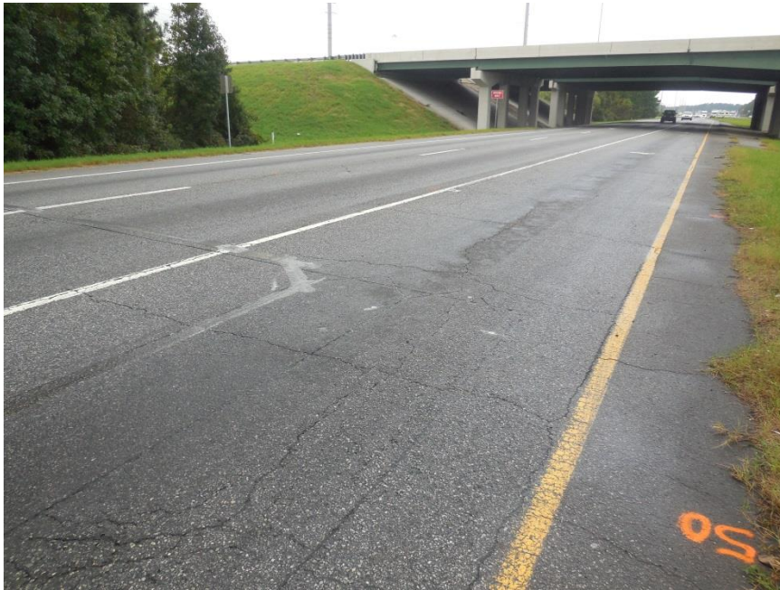
(13) Before- SR 25 NB @ I-95 left turn lane (7) facing SB
